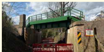
THE NEWLY INSTALLED BRIDGE.
