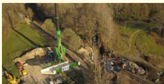
THE NEW BRIDGE GOING IN.
