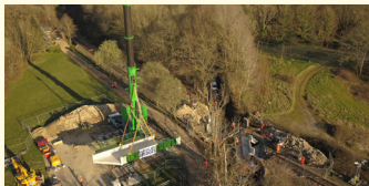
THE NEW BRIDGE GOING IN.
