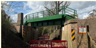
THE NEWLY INSTALLED BRIDGE.
